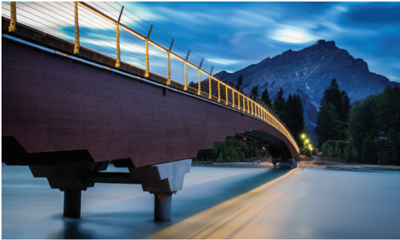
Bow River Bridge, Benff, Alberta (출처 : WoodWorks! BC)
